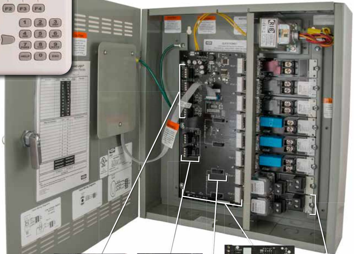
Load:Logic® 8-Relay Panel Interior
